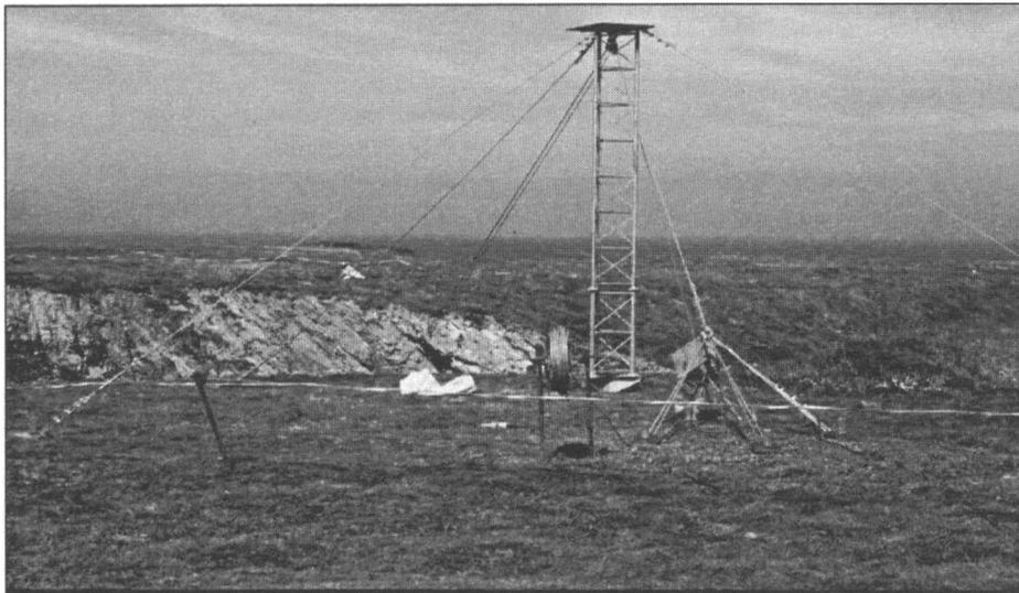
Illustration 3. Hoisting gear : tyrolean traverse.
